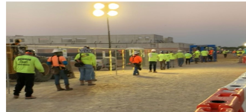
Workers keeping distant upon entry to site
